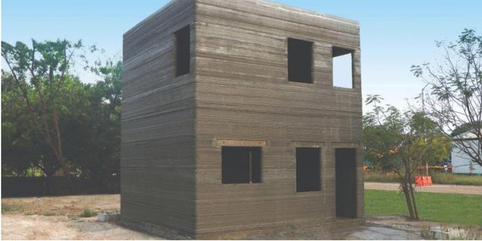
India's first 3D printed ground plus one-floor building with reinforcement has been constructed in Kanchipuram. The 3D printed building, a Ground plus one-floor building of 700 square feet built-up area, is constructed at Larsen and Toubro's Kanchipuram facility with a special, in-house developed concrete mix using indigenously available regular construction materials.
